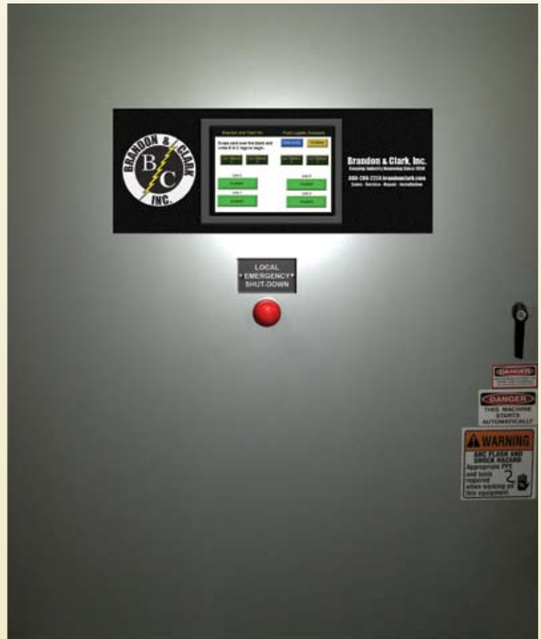
Station Control System Panel
